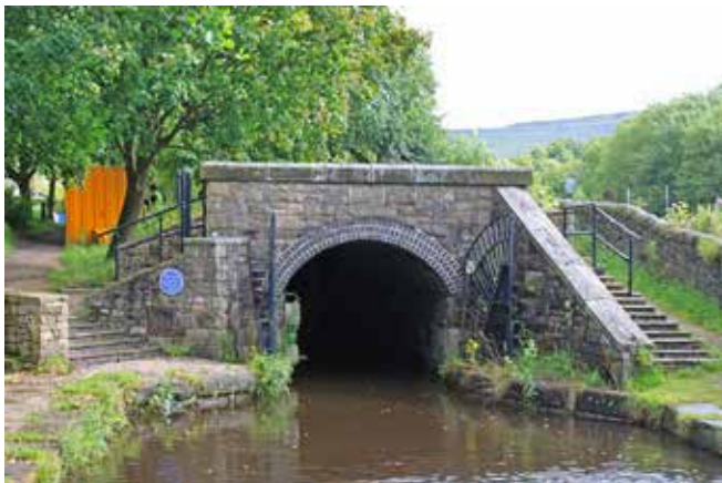
The Diggle portal
